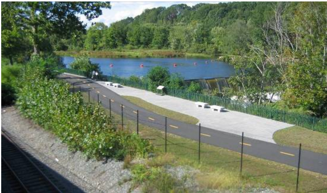
Figure 3.8: Blackstone River Bikeway and Manville Dam
