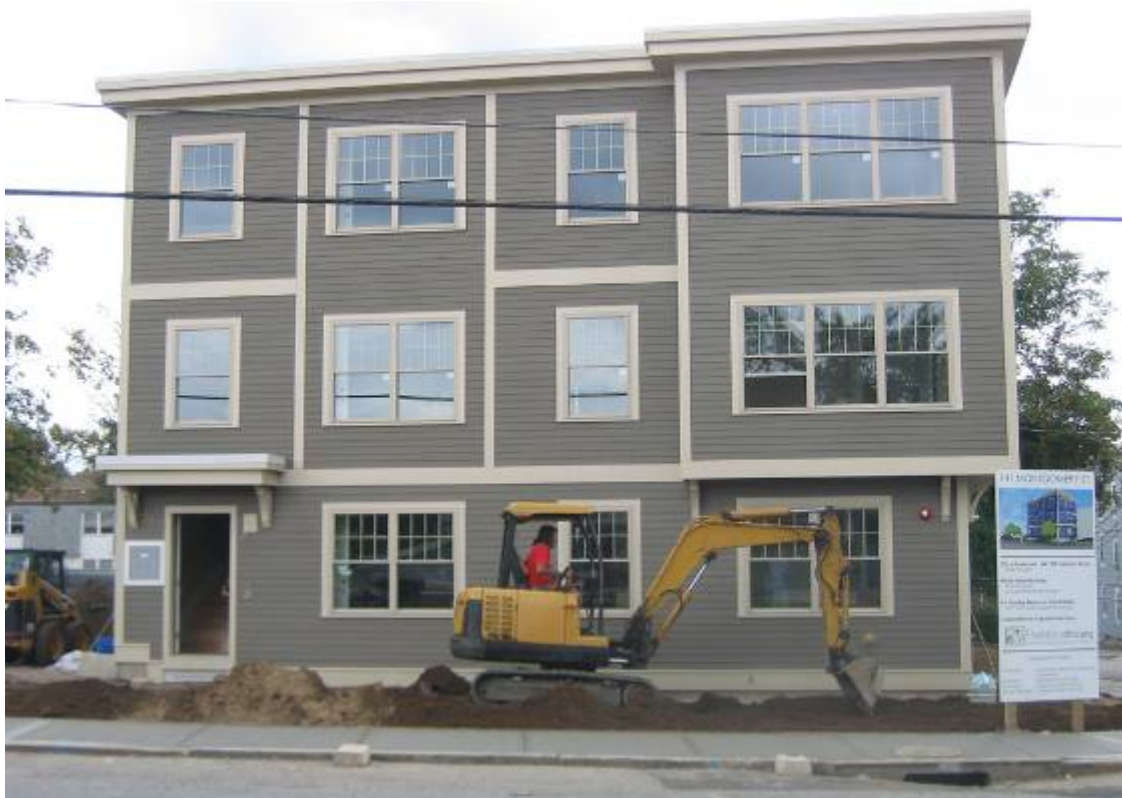
Figure 3.16: Townhouses under construction
