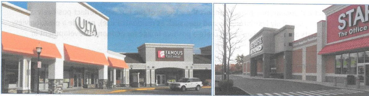
Figure 2: Varied roof lines and heights and a covered walkway with pedestrian scale ornamental lighting create a welcoming retail environment on the left. Varied façade treatments, column/articulation, and parapets provide
