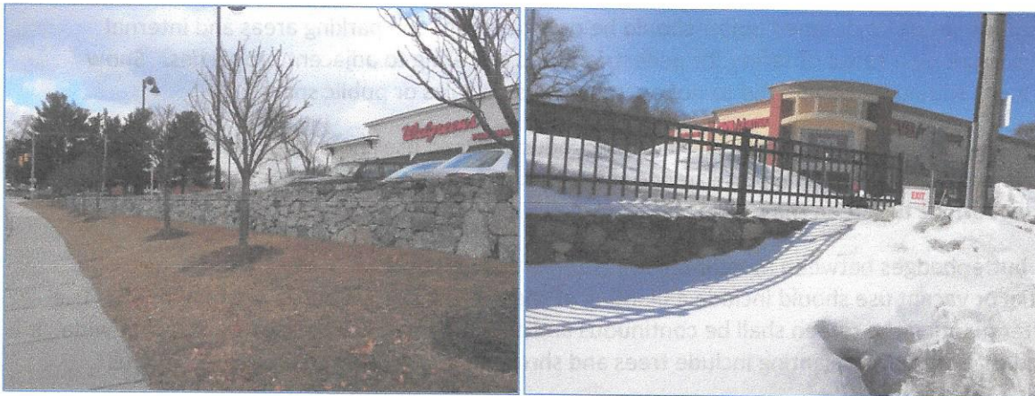
Figure 14: On the left, stone wall and street trees within the buffer zone to the rear of the sidewalk help incorporate a grade change and reduce the visibility of cars in parking lot. Ornamental metal fence and stone wall on the right separate the public and private realm and help divert attention of motorists and pedestrians from the parking lot to the rear of the fence (and snow).
