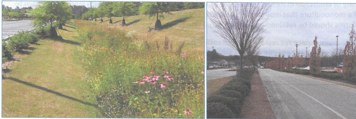
Figure 11: On left, bioretention garden helps manage stormwater flow from an adjacent parking lot. 6 On right, a progression of deciduous trees and evergreen shrubs line access road and provide four-season interest.
