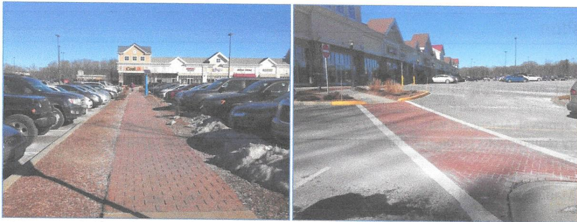
Figure 7: Paved path through parking lot and colored/textured crosswalks (stamped concrete) enhance pedestrian safety and encourage walking between shops. Note that sufficient snow storage area must be designated to enable four-season use of the pedestrian walkway.
