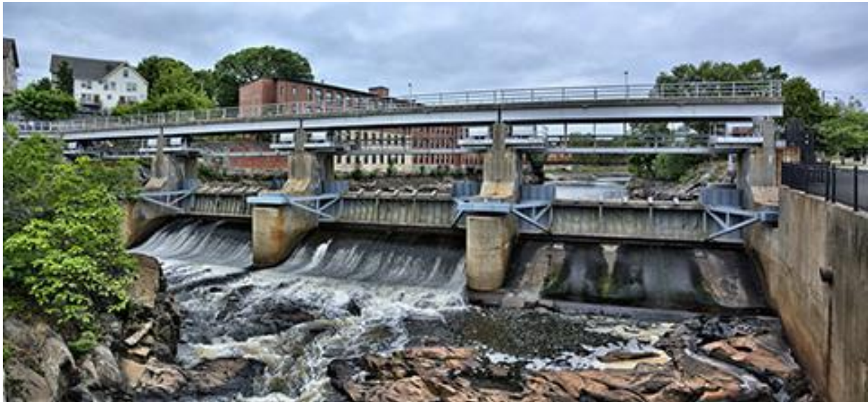
Thundermist Hydroelectric Plant (US Army Corps of Engineers)
