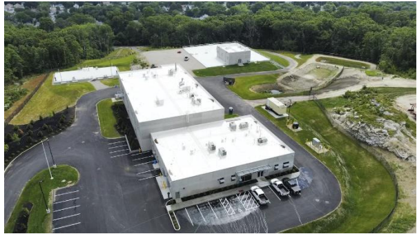
Woonsocket Water Treatment Plant (New England Construction)
