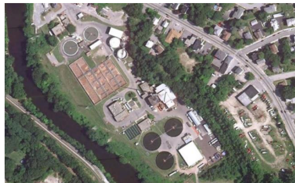
Woonsocket Regional Wastewater Treatment Facility (Google Earth)
