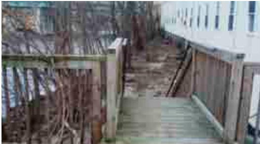
Floodplain and Parking
