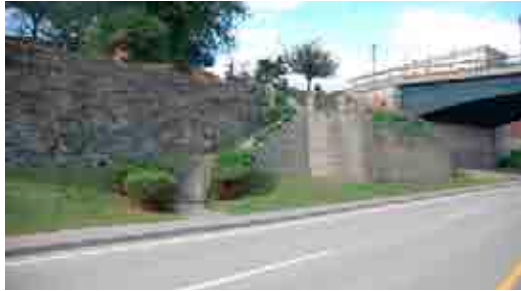
Existing Veterans Park Stairway
