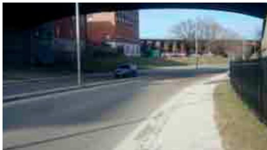
Court Street Bridge
